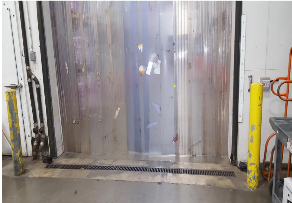
Photograph 17: View of drain outside of “Ice Box”.
