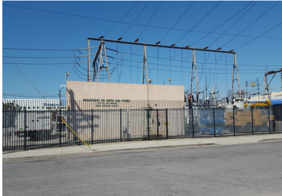
Photograph 7: View of the eastern side of the LADWP generation station.
